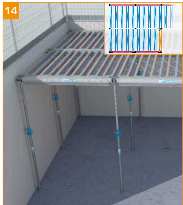
- Continue to mount the C2+ progressively using the TopPerche, or C4+ frames from one to the next.
